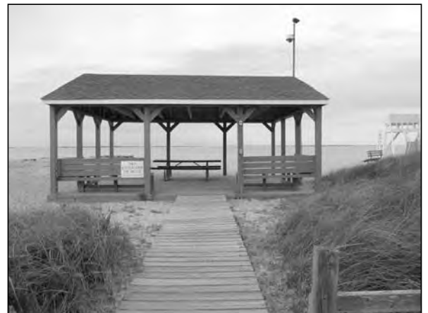
New electric outlets and lighting
