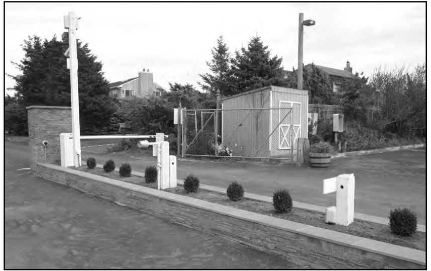
The new stone planters
